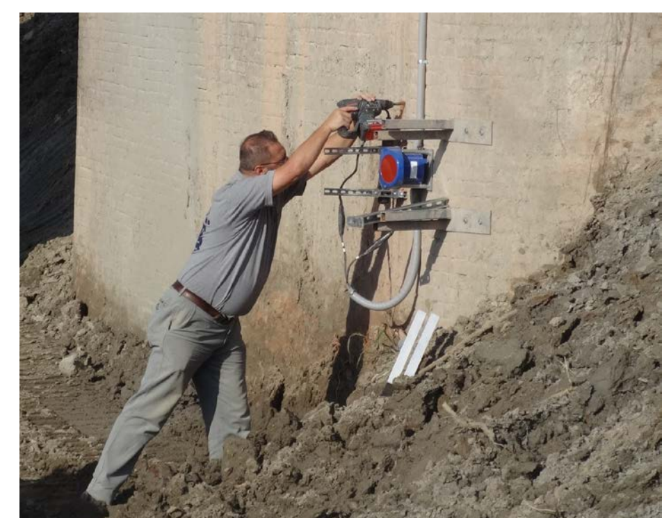
The Secchia river (Italy) at Motta bridge with an outline H-ADCP profiling (left). Instrument installation at bridge pier (right) during dry period.
