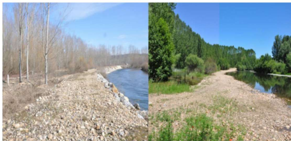
Figure 4. River bank protections were also removed along the river: on the left, the situation before the project; on the right, the river is reconnected to its floodplain (source: Duero River Basin Authority – Confederación Hidrográfica del Duero, CHD).
