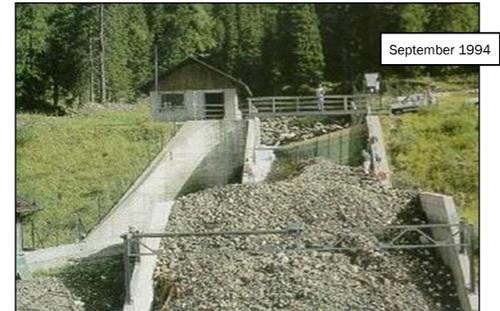
Fig. 2: Bedload material transported by September 1994 event
